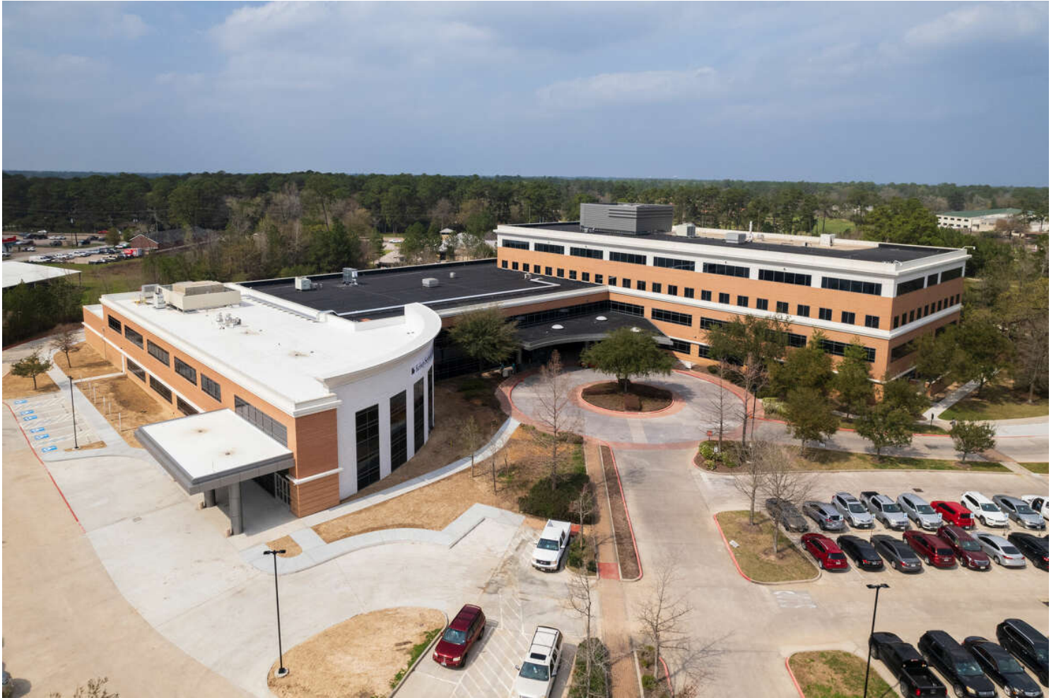
Kelsey-Seybold Clinic - Spring Medical and Diagnostic Center at 15655 Cypress Woods Medical Drive now totals 172,000 square feet after a 12,000-square-foot expansion on the first floor and a 28,000-square-foot addition on the south side of the building.
